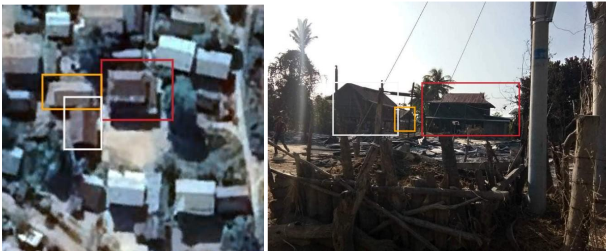
Figure 41: Geolocation of burned houses and destruction in Yae Myet village.
