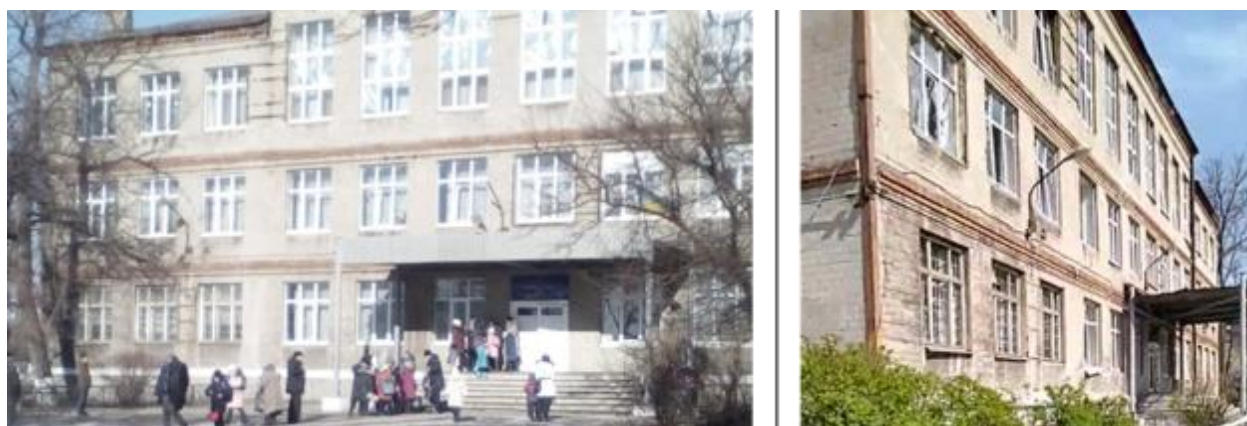
Figure 22: School #24 before (left) and after (right) damage
