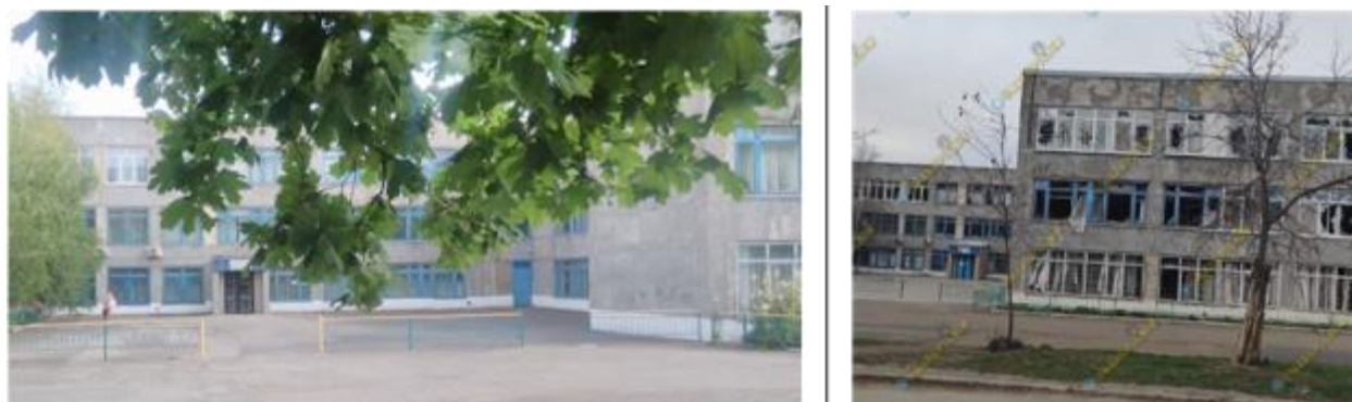
Figure 38: School #41 before (left) and after (right) damage
