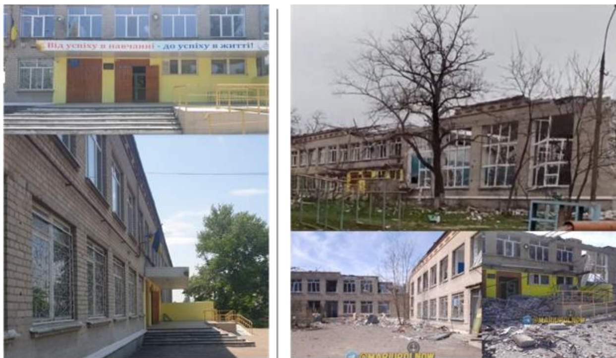
Figure 40: School #57 before (left) and after (right) destruction
