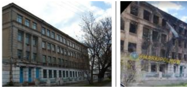
Figure 32: School #37 before (left) and after (right) damage
