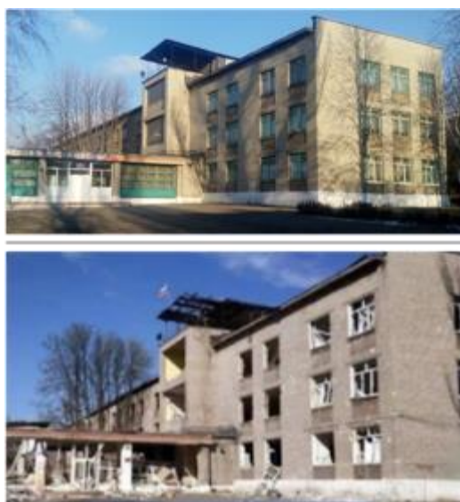
Figure 33: School #54 before (top) and after (bottom) damage
