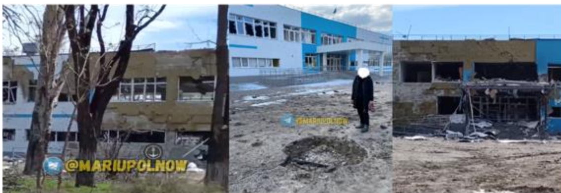
Figure 28: Before (top) and after (bottom) the damage to school #15 in Mariupol
