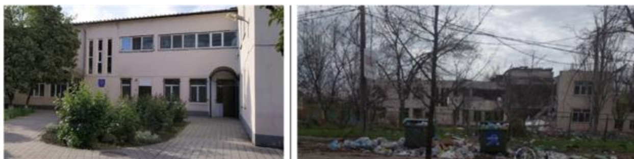
Figure 25: Kindergarten #167 before (left) and after (right) damage.
