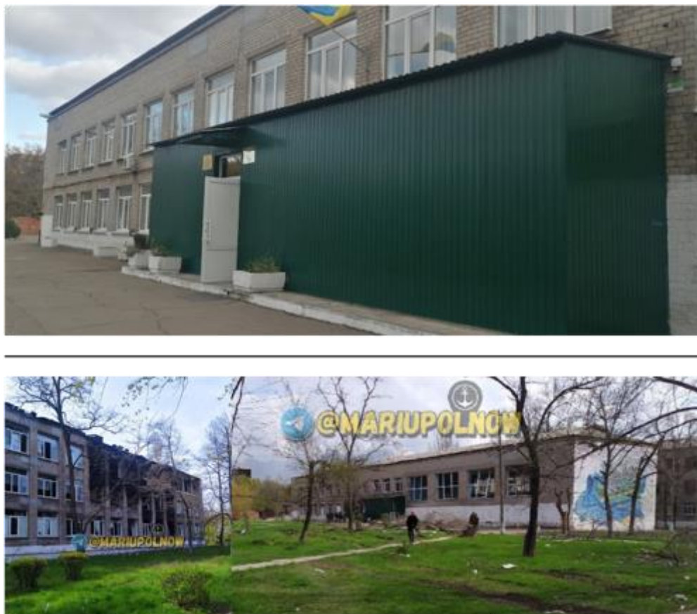
Figure 10: School #9 before (top) and after (bottom) damage
