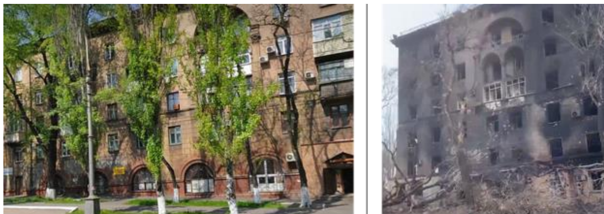
Figure 18: Before (left) and after (right) heavily damaged art school
