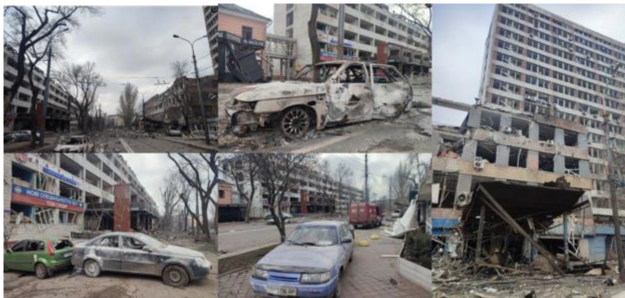
Figure 4a: Images of the destroyed Pryazovskyi State Technical University building and its surroundings
