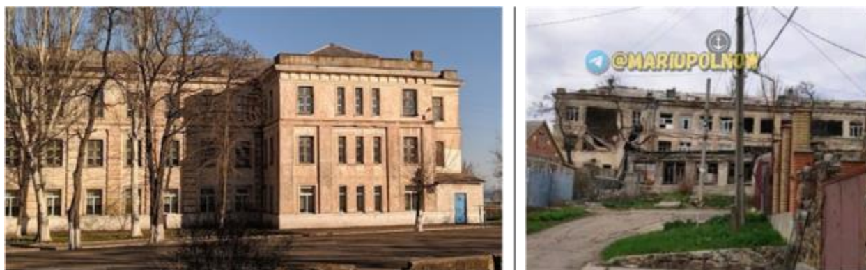
Figure 30: School #32 before (left) and after (right) damage
