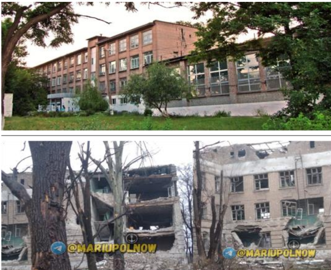
Figure 24: School #45 before (top) and after (bottom) damage.
