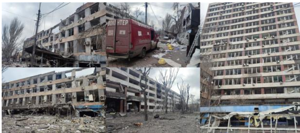
Figure 4b: Images of the destroyed Pryazovskyi State Technical University building and its surroundings
