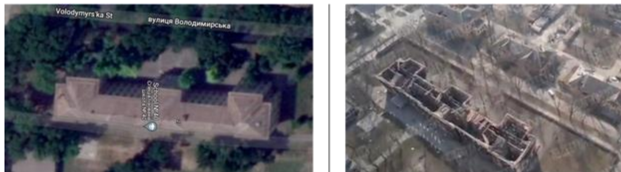
Figure 37: Satellite image of the school (left) and the drone footage of the collapsed roof (right)
