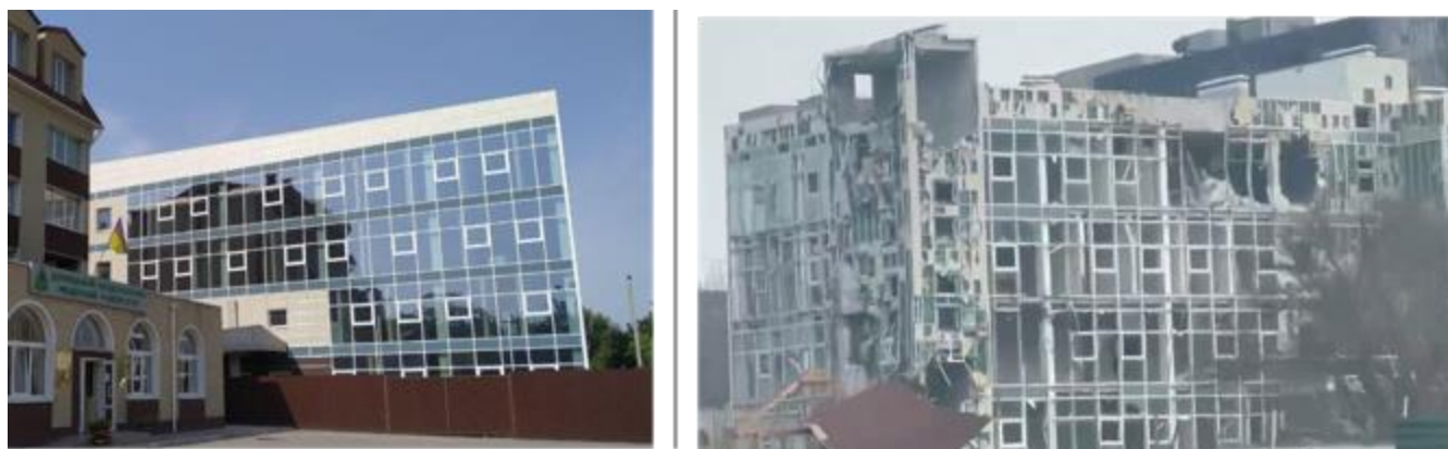
Figure 9: Medical Institute before (left) and after (right) destruction
