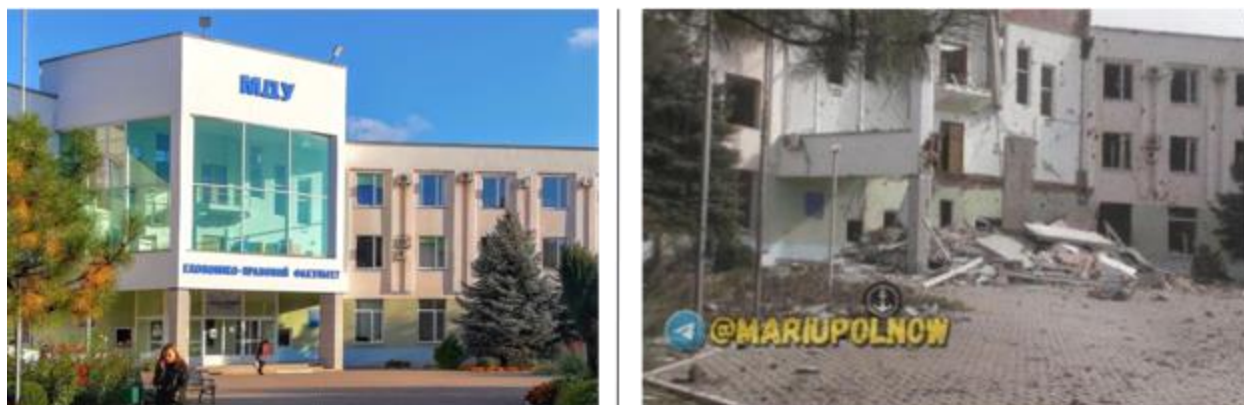
Figure 6: Faculty of Economics and Law of Mariupol State Humanitarian University before (left) and after (right) destruction
