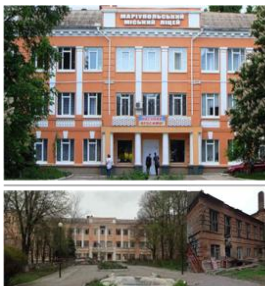
Figure 17: Mariupol City Lyceum before (top) and after (bottom) damage
