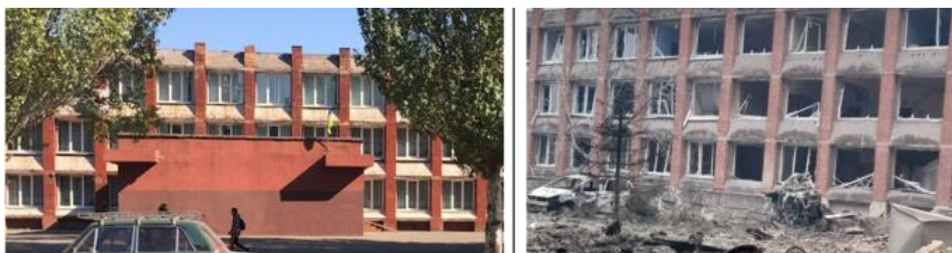
Figure 8: College before (left) and after (right) damage
