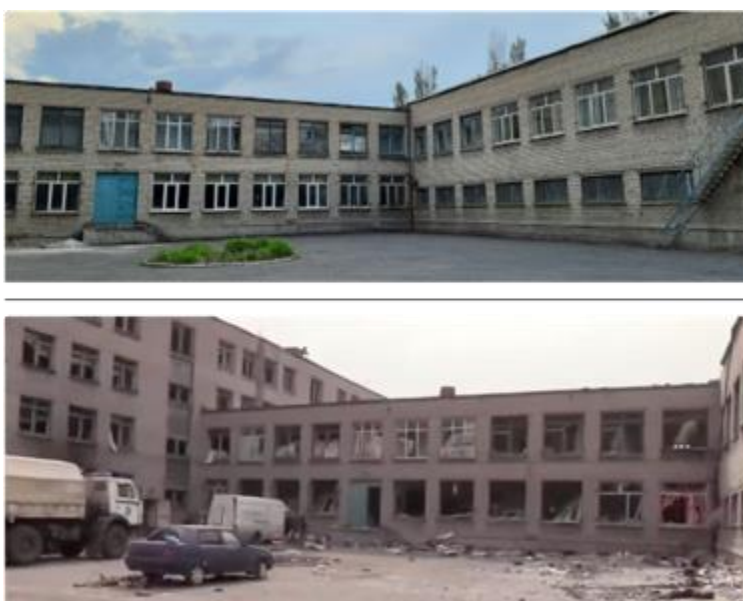
Figure 11: School #25 before (top) and after (bottom) damage
