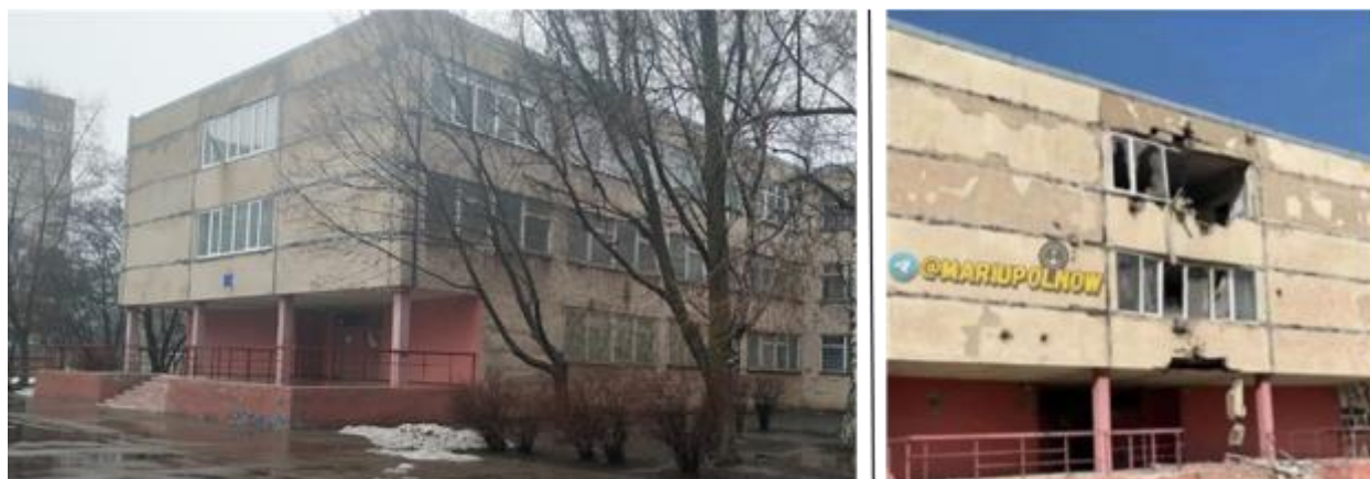
Figure 16: School #67 before (left) and after (right) damage
