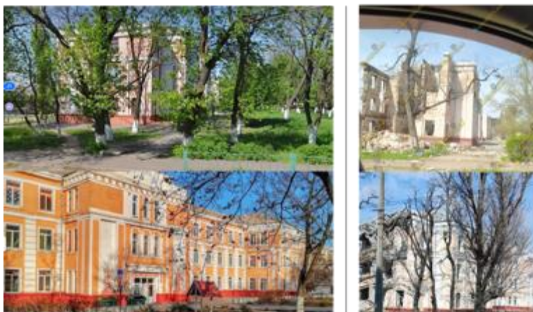
Figure 12: Before (left) and after (right) the damage to school #36 in Mariupol
