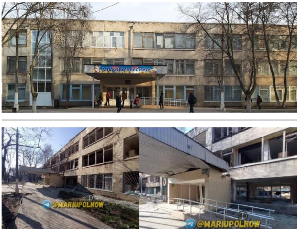
Figure 13: School #52 before (top) and after (bottom) damage
