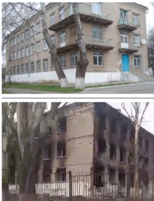
Figure 35: School #2 before (top) and after (bottom) damage
