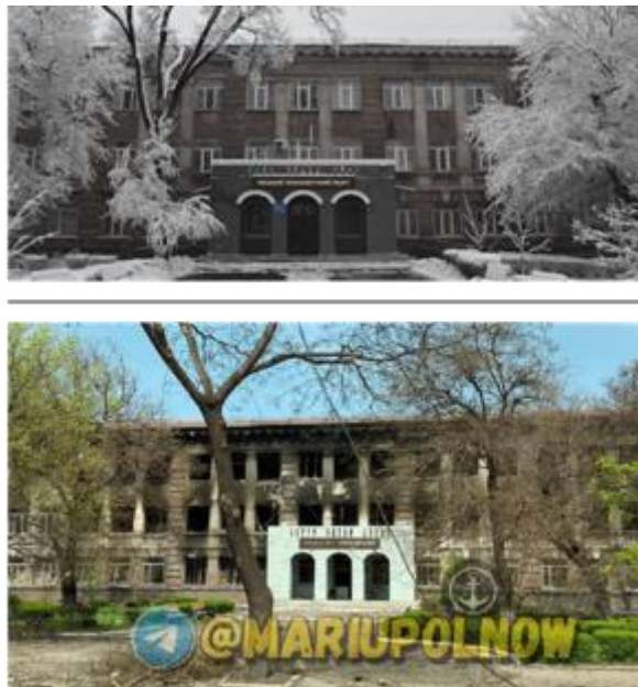
Figure 26: Technological Lyceum before (top) and after (bottom) damage.
