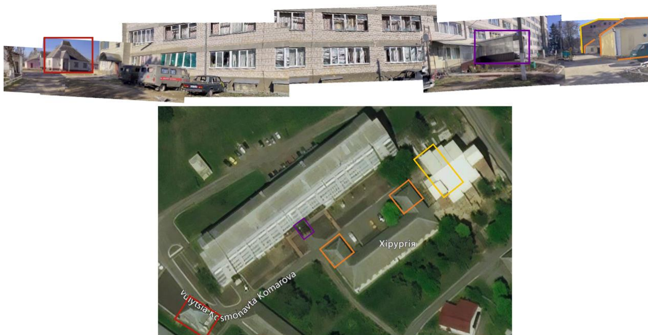
Figure 9: Geolocation of footage showing damage to Makariv's Hospital.
