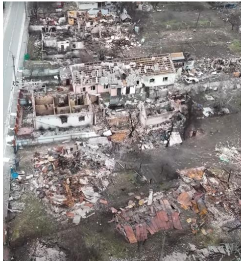
Figure 19: A Screenshot of drone footage showing the destruction of residential buildings.
