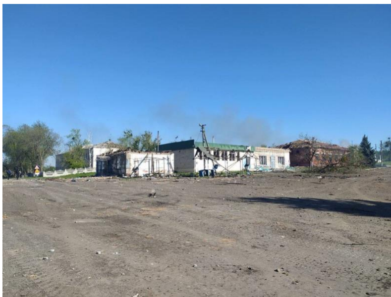
Figure 12: Footage from 14 May, showing civilian infrastructure destruction in Shandryholove, Donetsk Oblast; geolocated to 49.102042, 37.715111.
