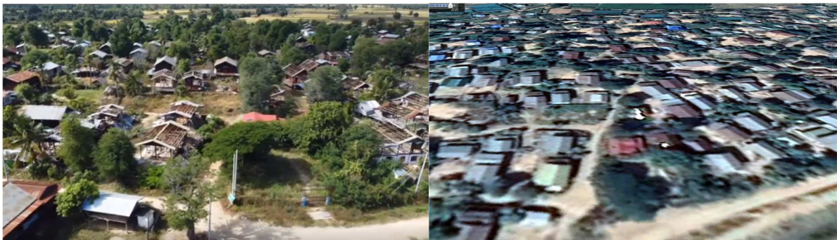
Figure 37: Geolocation of damage through drone footage of Kar Paung Kya (ကာပေါင်းကျ) at 23.091879, 95.273063. Satellite imagery from Google Earth.
