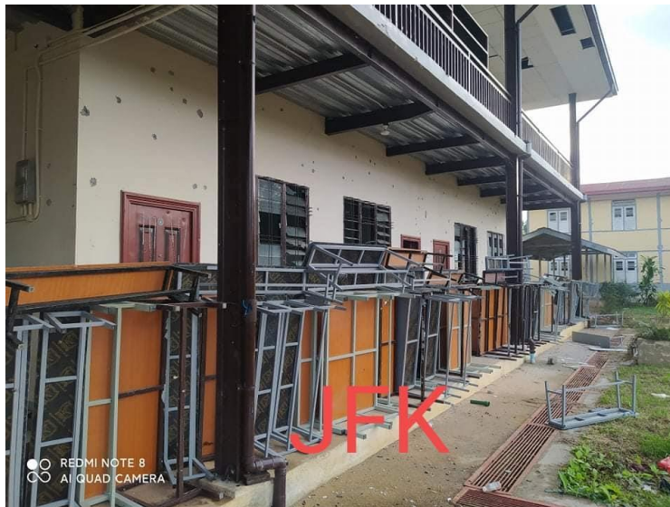
Figure 15: Barricaded building in Moe Bye (မိုးဗြဲမြို့) [19.740617, 97.091802], shared online on 13 September 2022 (Source: JFK Page 3 ).
